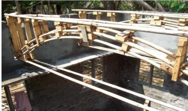
Fig. 5 : Twin Vertically Separated Bamboo bows With Wooden Spacers to take roof loads
