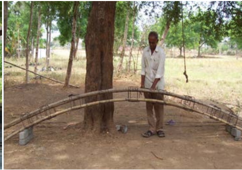
d) Bow Beams with Steel Ties
