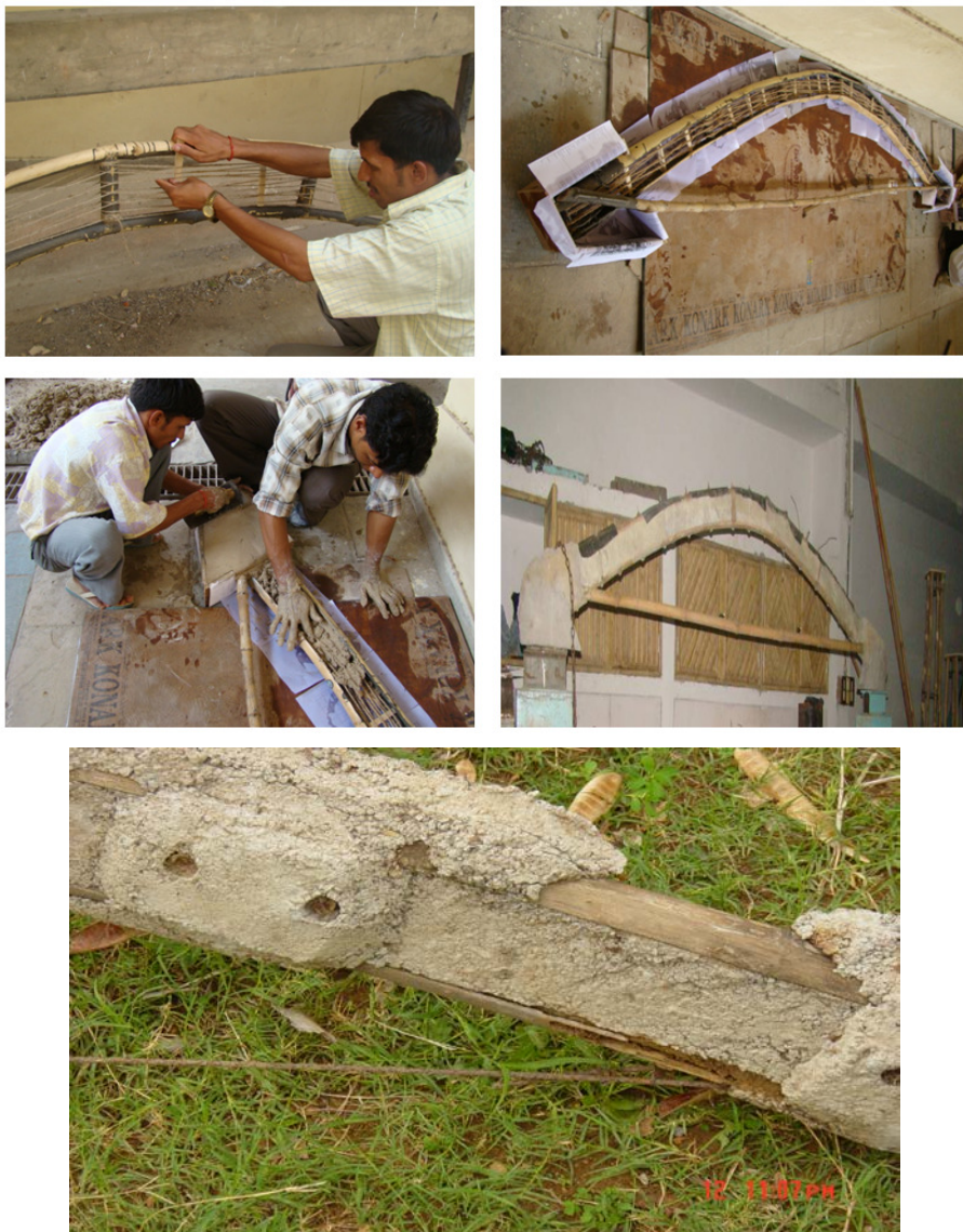
Fig. 14 Construction of a infilled half split bamcrete arch
