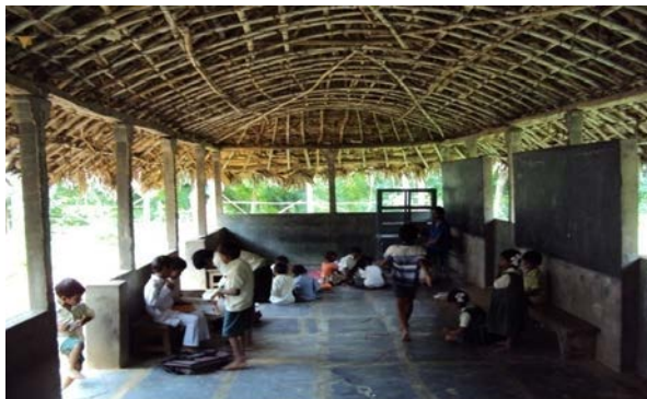
Fig. 2 A Frame Structure with Thatched roof for class room
