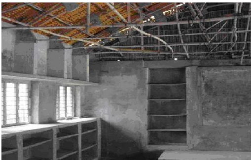
e) Inside View – 7.3 m Structure
