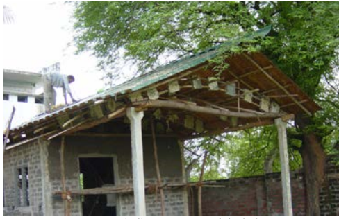
a) Structures with 3.3 m span
