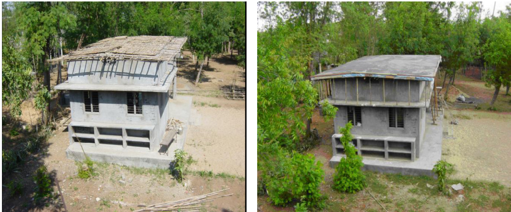
Fig. 6: Bamboo House with Bamboo roof panel before putting on Cellular concrete
